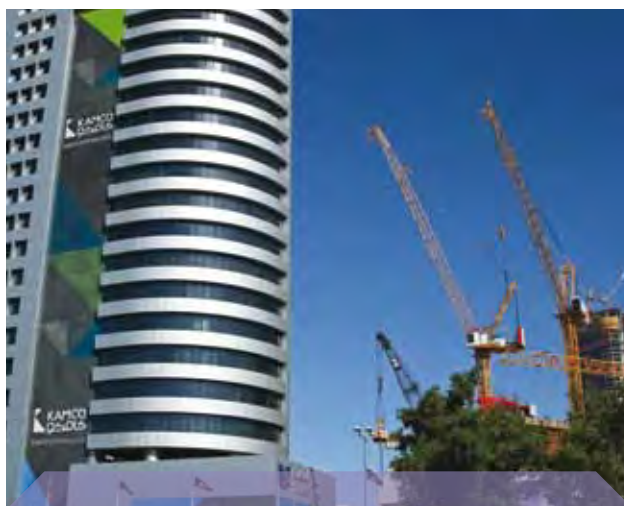
Kuwait City: skyscraper under construction.
