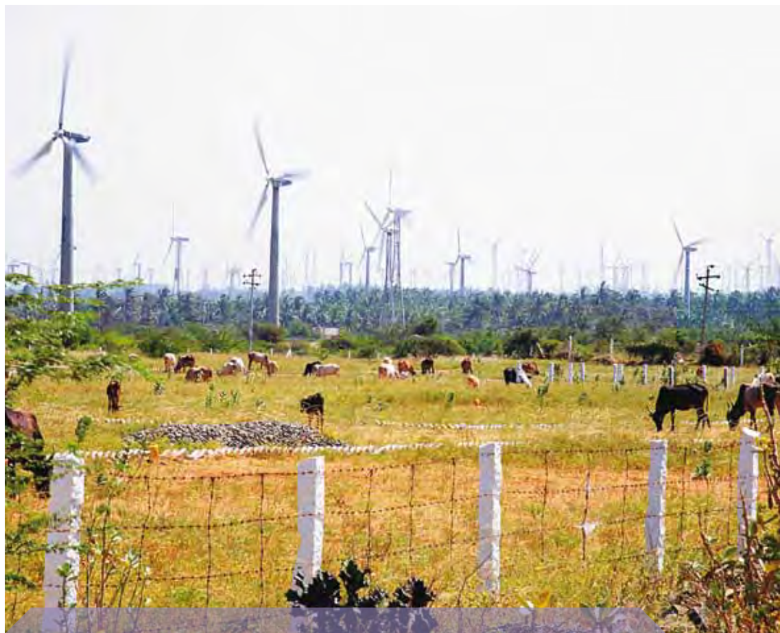
India: the wind turbine area of southern Tamil Nadu runs for mile after mile across the plains south of the Southern Ghats mountains, producing electricity for part of the massive demand for power throughout India.
