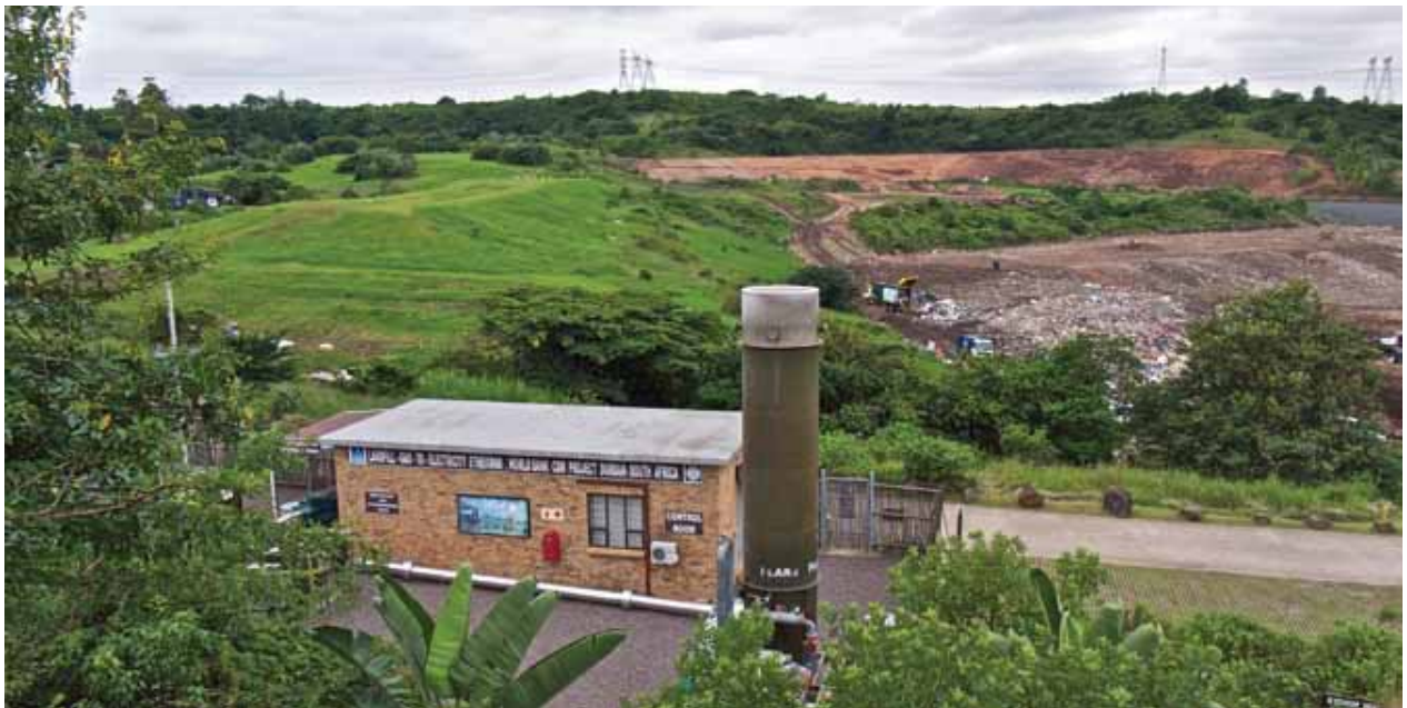
▲ The Marianhill Landfill Conservancy is a unique initiative by the eThekweni Municipal Area (EMA) that is both a waste disposal site and an area of natural beauty. Top: Photo courtesy of Landfillconservancies.com Bottom: ©BBC World Service. Licensed under the Creative Commons Attribution-NonCommercial 2.0 Generic License.
