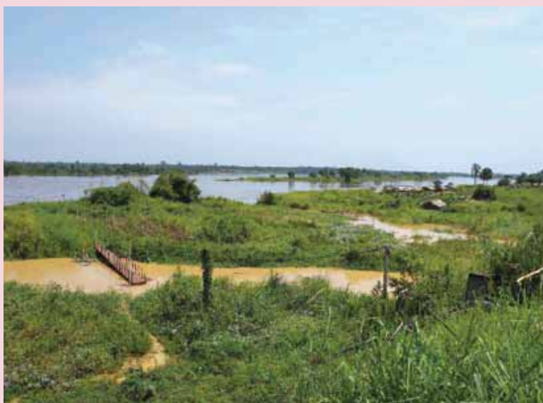
▲ Degradation of the catchment supplying the public water utility's (REGIDESO) treatment plant in Kindu is threatening its operation. ©UNEP
