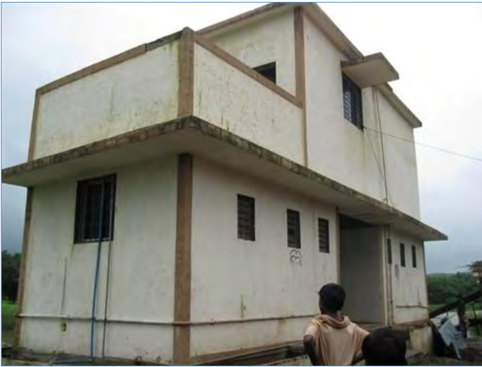
A new toilet block constructed in Karjat near Mumbai after an old toilet block was demolished. Photo: SPARC
