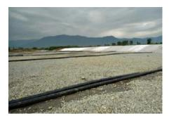
The underground drainage system for leachate collection
