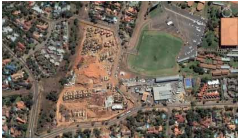
The site under construction
