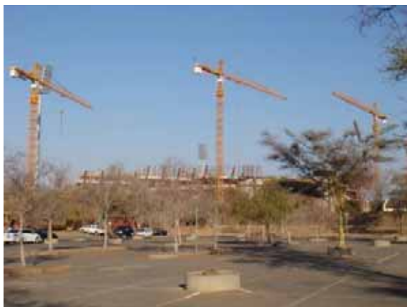
Construction at the stadium
