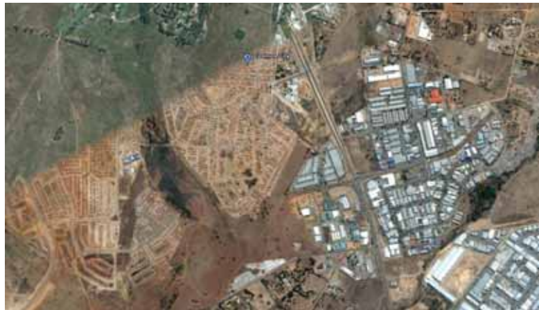
The site under construction
