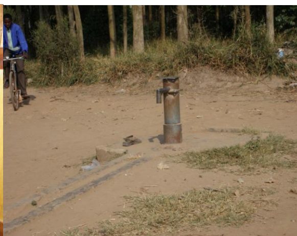
Non-functioning water pump.
