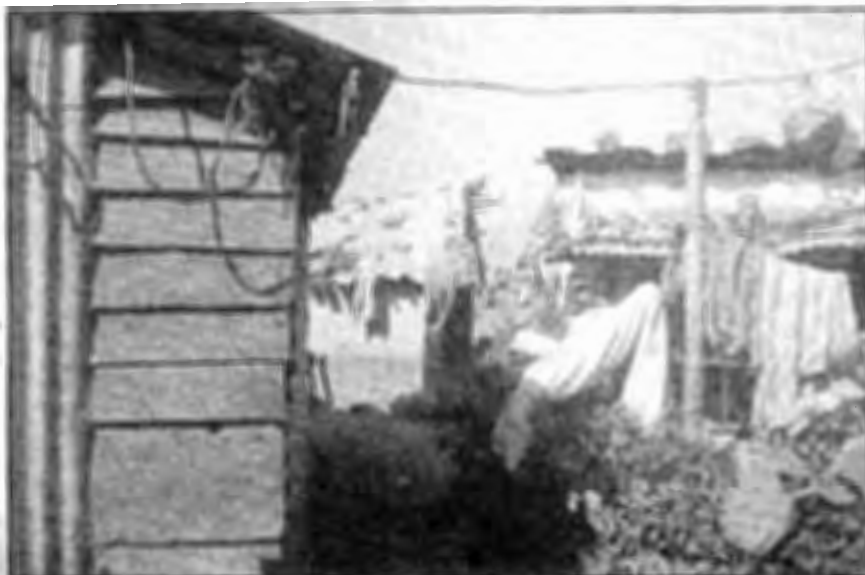
A Typical Condition of Squatter House
