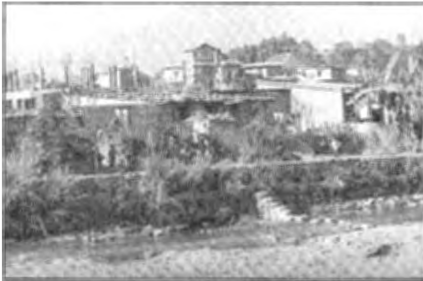
Typical Settlement along Riverside
