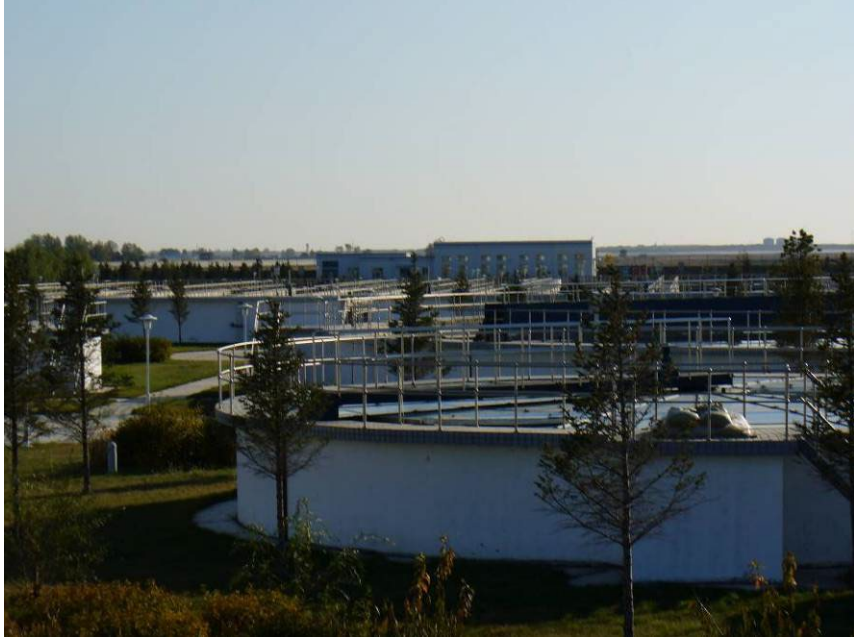
Main building and treatment units at Qiqihar Number 1 Wastewater Treatment Facility
