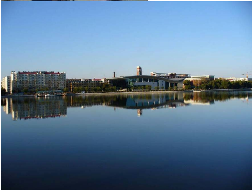
Intake line and pump station feeding Labour Lake from Nenjiang River. Final picture is portion of Labour Lake already completed at University.
