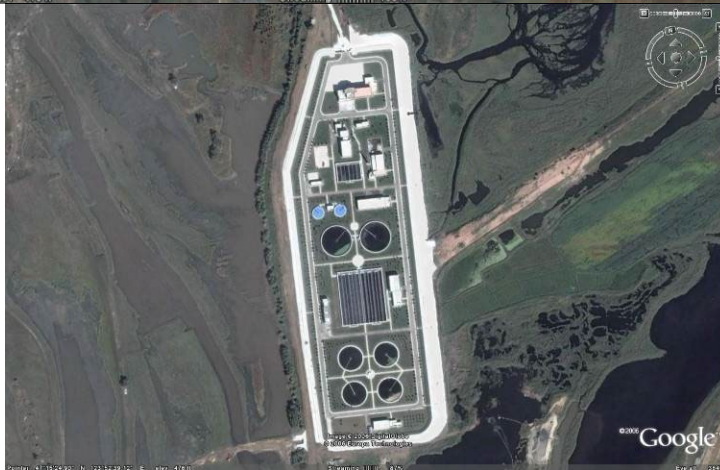
WWTP1 (WWTP2 proposed to be on right, reuse plant below)
