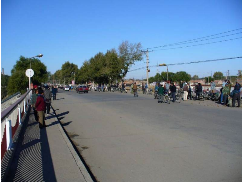
South End of Phase 2 Labour Lake Project looking north. This is major bridge replacement included in project, south end.
