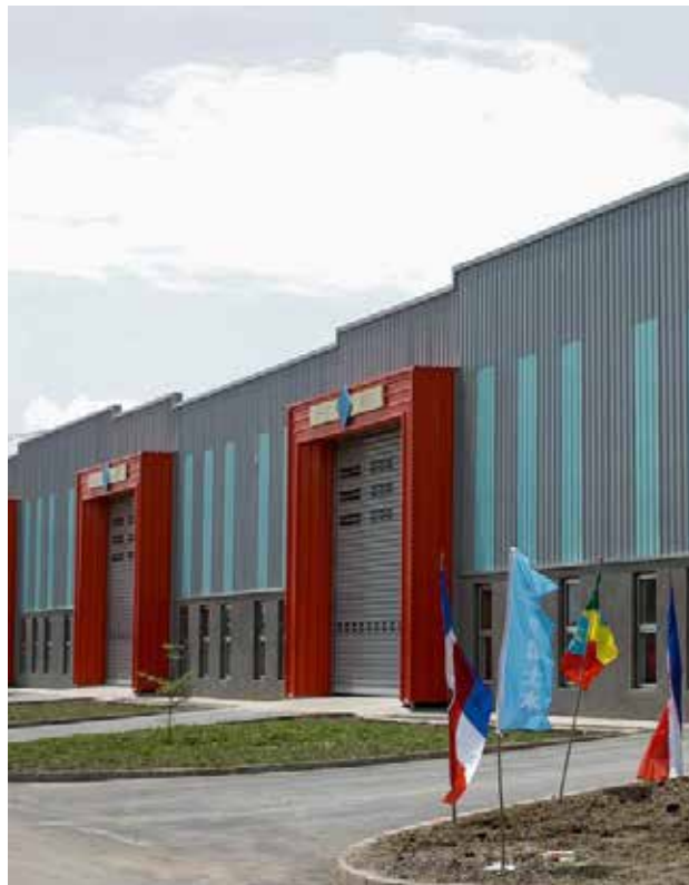
Hawassa Industrial Park.
