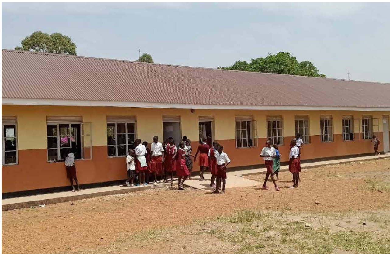
A four-classroom block in Koboko's Birijaku Primary School built through the Action.
