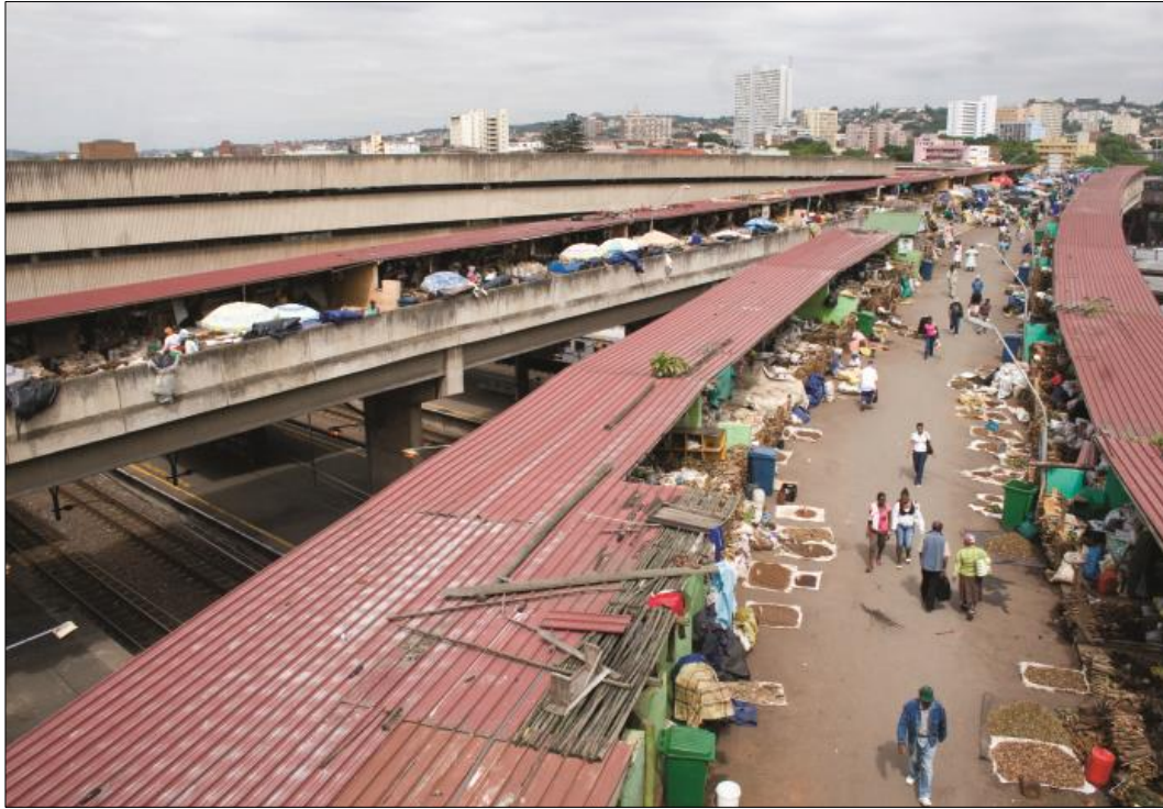
Figure 10.2: Ariel view, Herb Market, Warwick Junction (Source: The city at eye level, 2016)
