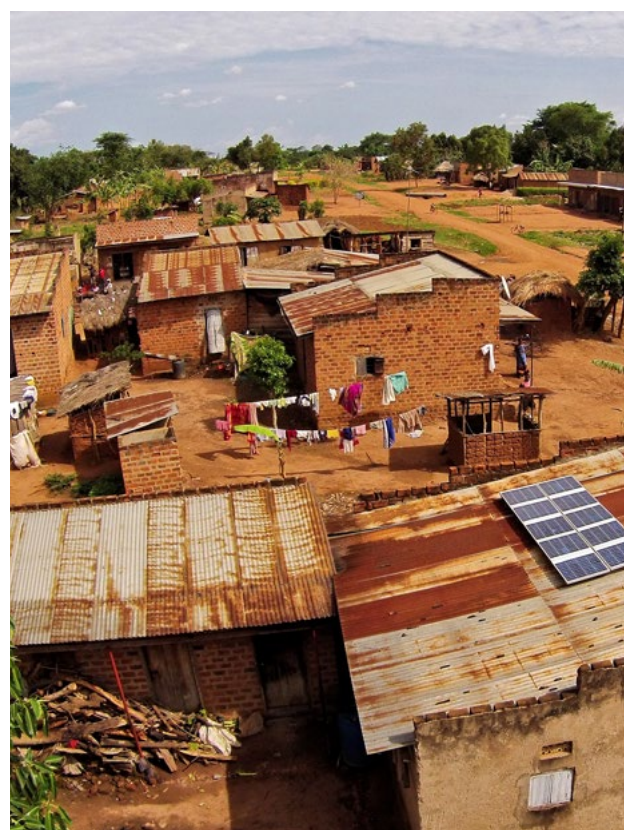
A residential solar system in Uganda deployed by SolarNow, one of SunFunder's customers. (Photo: SunFunder)
