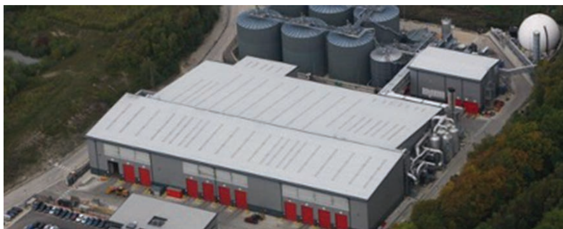
FIGURE 16: Biffa/West Sussex Mechanical Biological Treatment Plant, rated for 100,000 tonnes per year of organic waste (310,000 tonnes per year of MSW)
