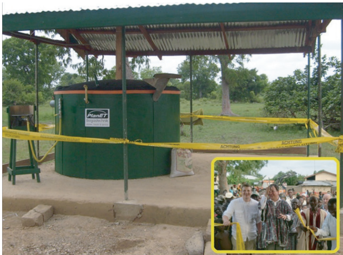
FIGURE 78: Micro-scale digester installed in Ghana by PlanET Biogas Solutions
