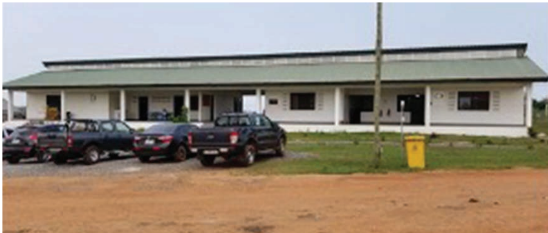
FIGURE 42: Safi Sana offices
