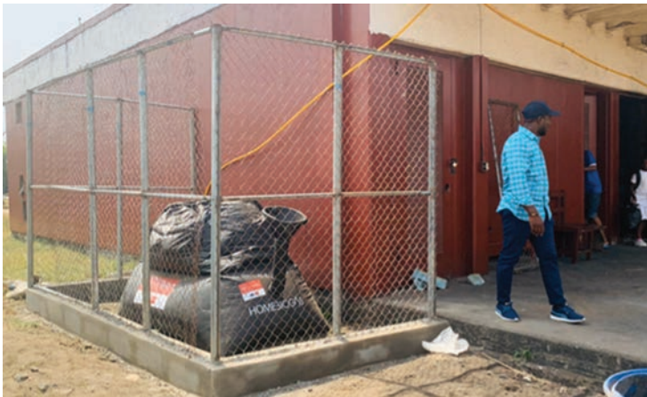
Example of fencing installed around the unit
