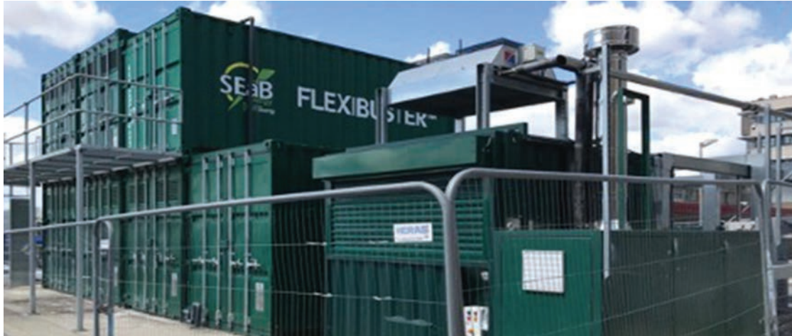
FIGURE 22: FlexiBuster installation at University Hospital in Southampton UK rated at 3 tonnes per day of waste food
