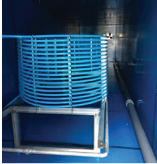
FIGURE 19: bioQUBE digester tank heating coil
