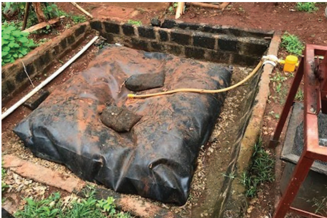
FIGURE 33: Sistema Bio very small-scale biogas system visited in Kenya
