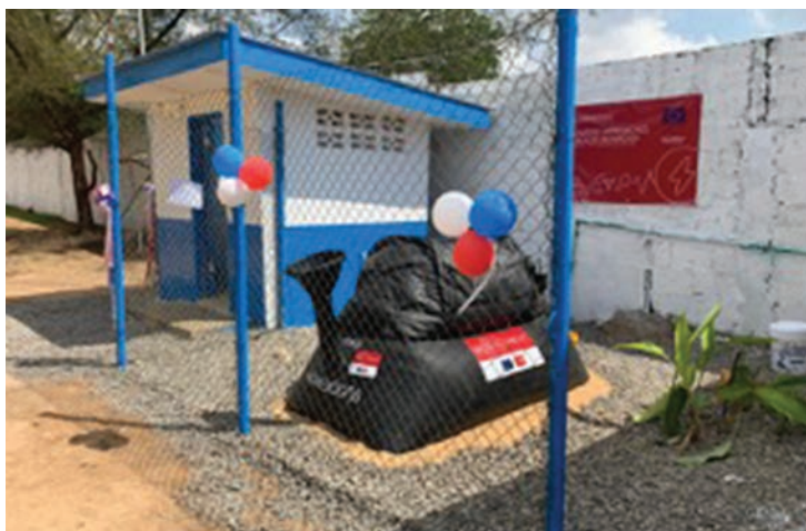
HomeBiogas unit and toilet facility prepared for the launch event
