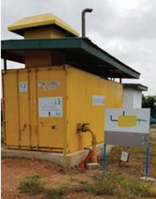
FIGURE 44: Power generation module
