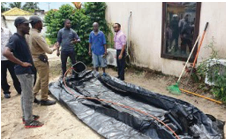
Installing 7.0 unit at RLJ Kedneja Hotel
