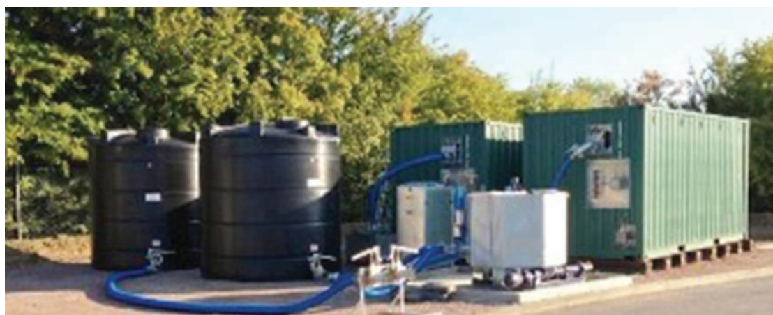
FIGURE 17: bioQube – A pre-packaged, modular, wet ad system with power generation
