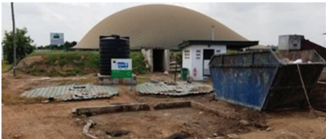
FIGURE 43: Primary anaerobic digester
