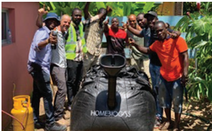
Installation of 2.0 unit at Tropicana Resort
