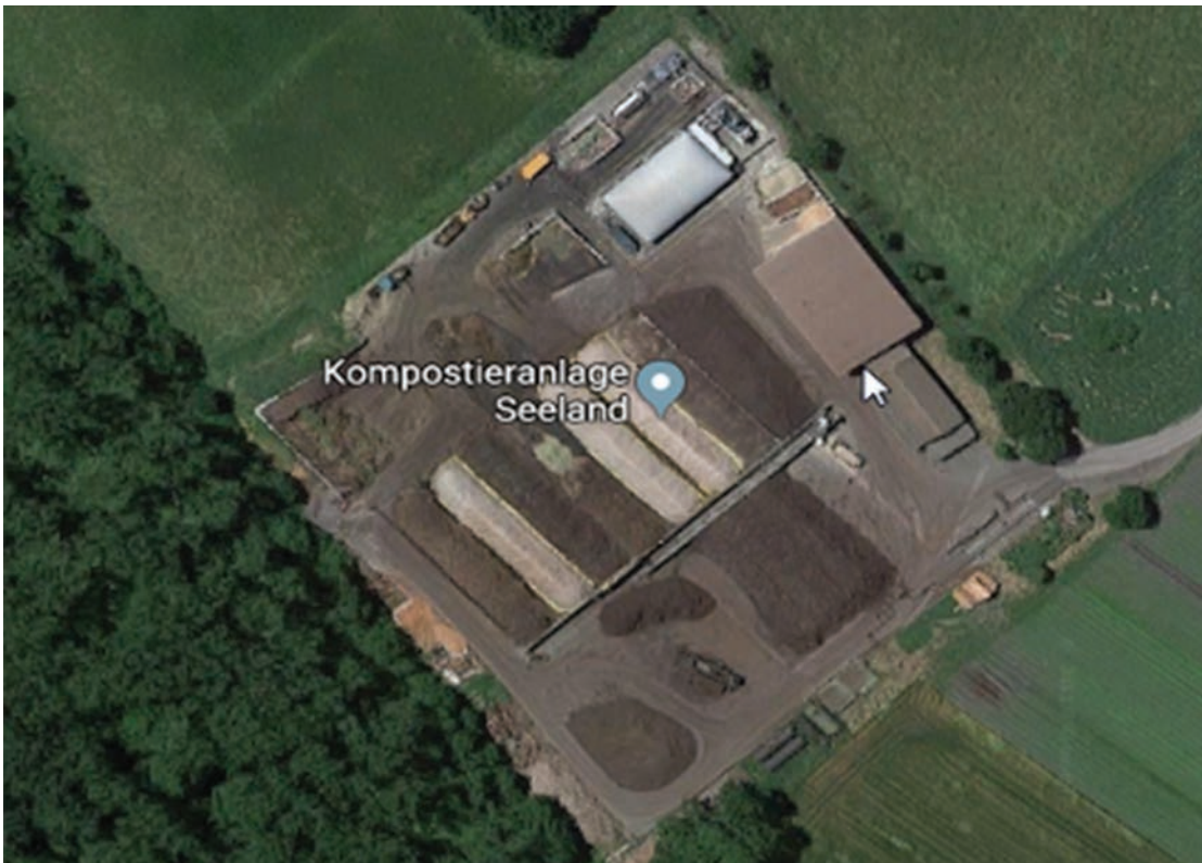
FIGURE 51: BEKON MINI installation in Switzerland rated at 4,500 tonnes/year of waste organics
