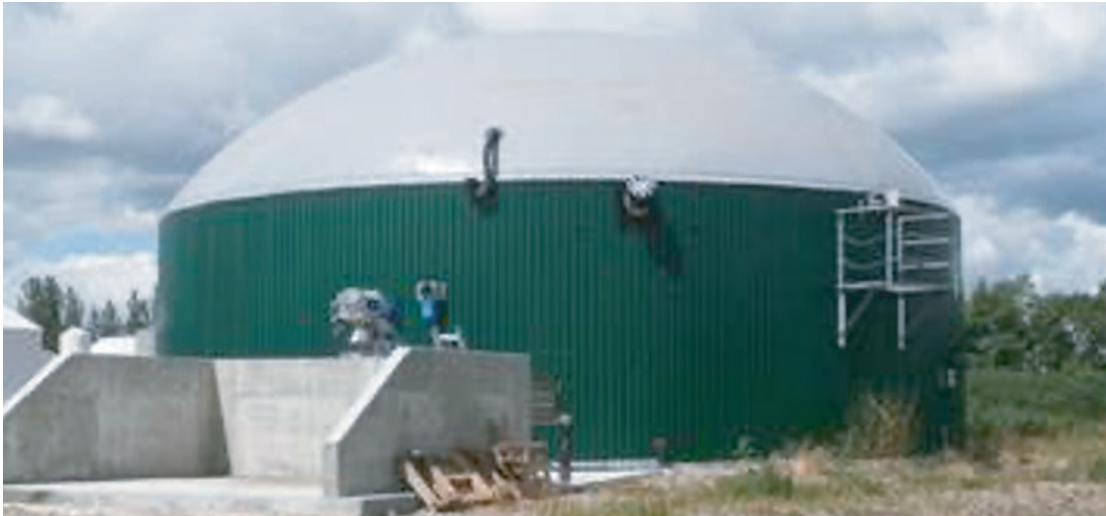
FIGURE 79: PlanET Biogas Solutions anaerobic digester
