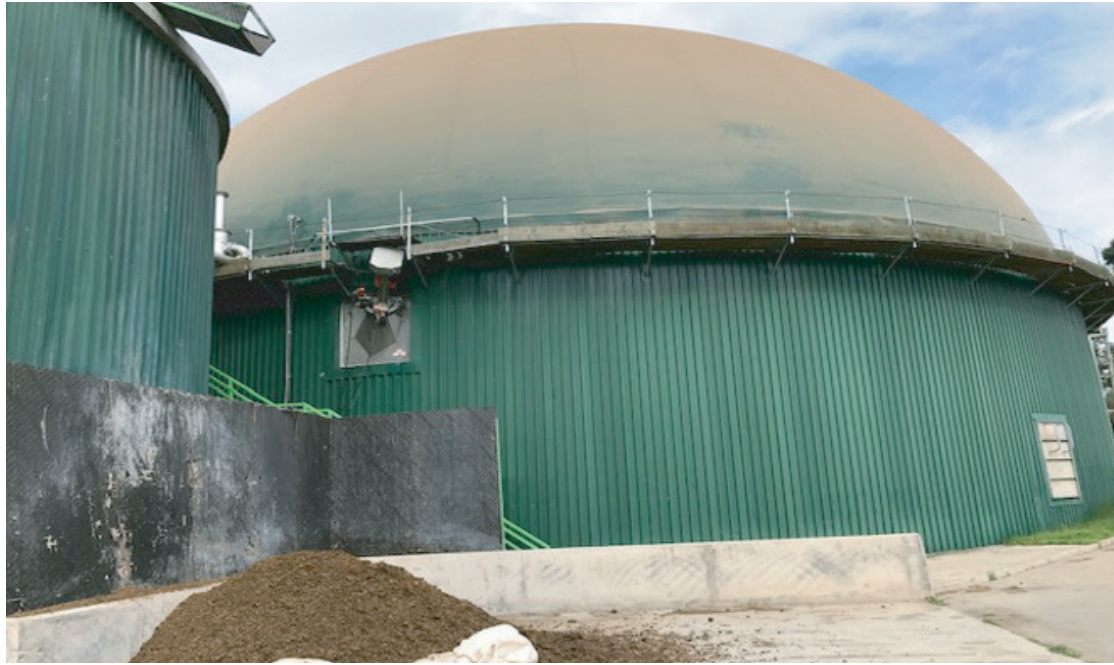
FIGURE 67: Example of digester (at Gorge Park Energy Farm Kenya)
