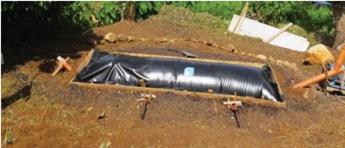
FIGURE 23: HoMethan installation in Grenada, Caribbean rated for 200 kg per day of manure slurry
