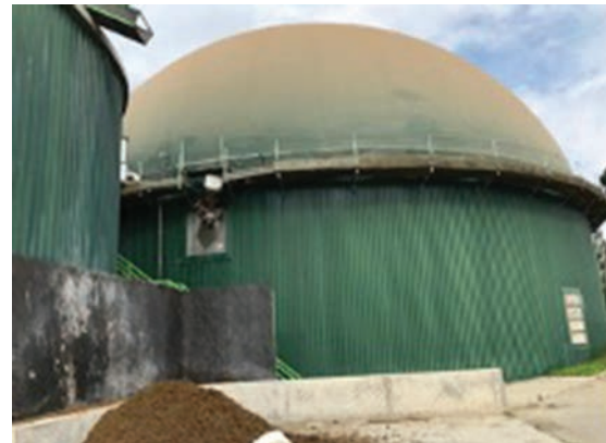
FIGURE 38: Primary anaerobic digester tank
