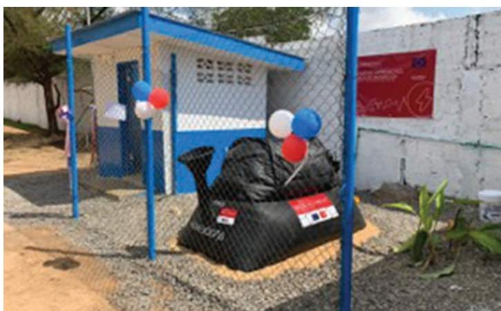
HomeBiogas unit and toilet facility prepared for the launch event at Isaac A. Davies School
