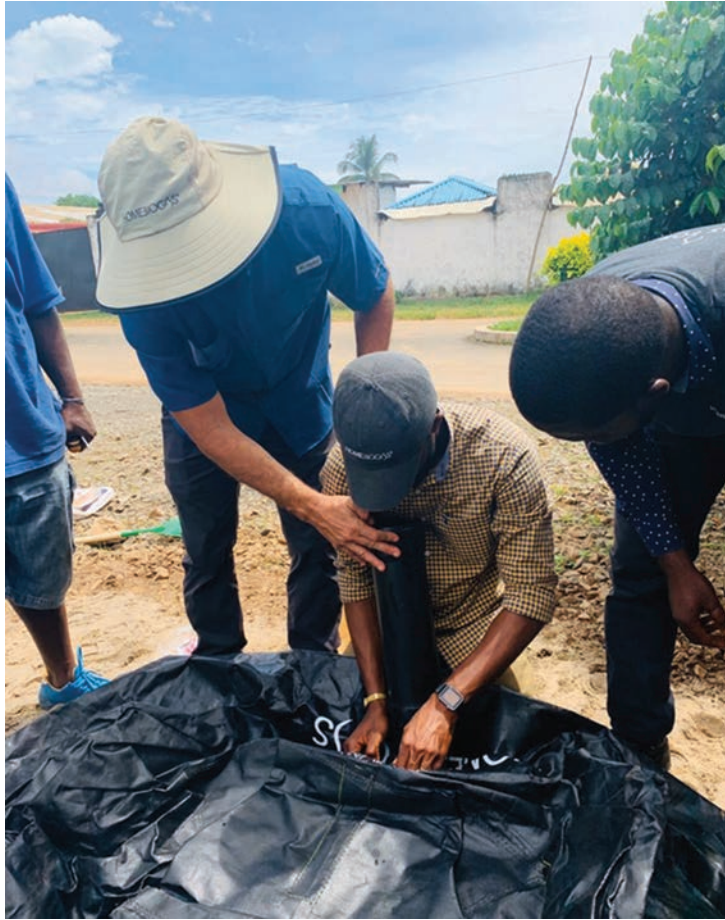
HomeBiogas personnel training WNL Local Coordinator Septimus Nyanforh on installation methods
