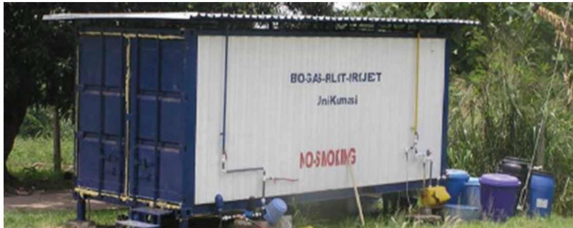
FIGURE 13: Experimental Dry Anaerobic Digester deployed at the University of Science and Technology (KNUST) in Kumasi, Ghana
