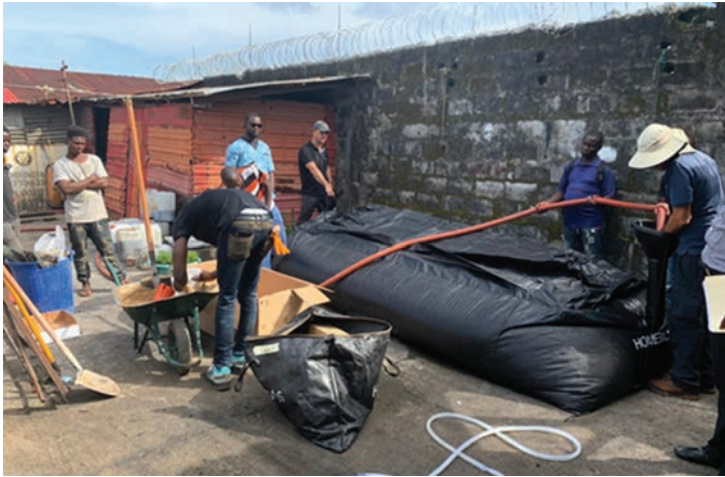
Installing 7.0 unit at Corina Hotel. Photo shows filling the unit with water.
