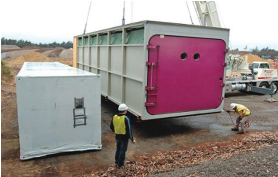
FIGURE 48: Dry-type AD modules permit easy scalability
