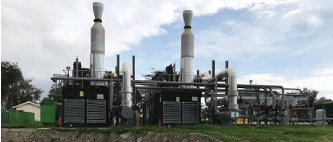
FIGURE 39: Biogas power generation facility
