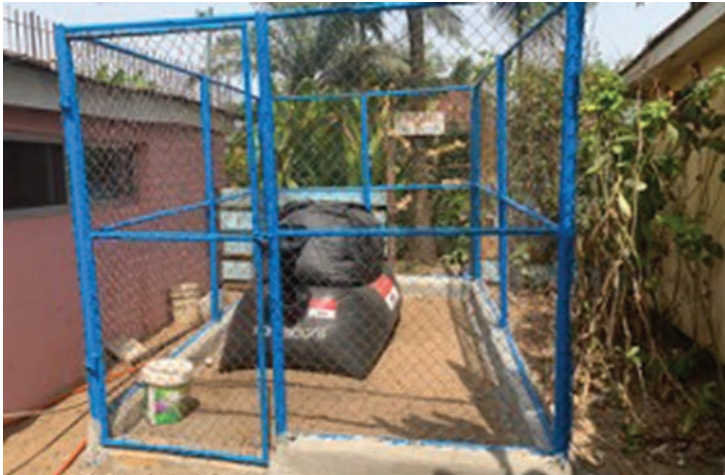
Fence installed at Tropicana Resort
