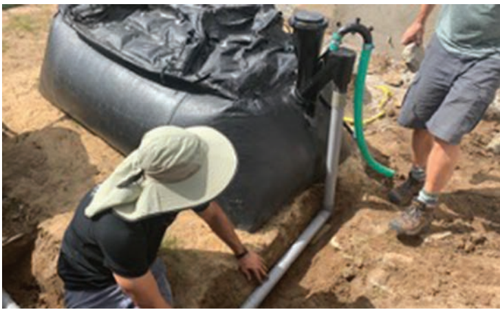
Installing piping for HomeBiogas toilet at Isaac A Davies School
