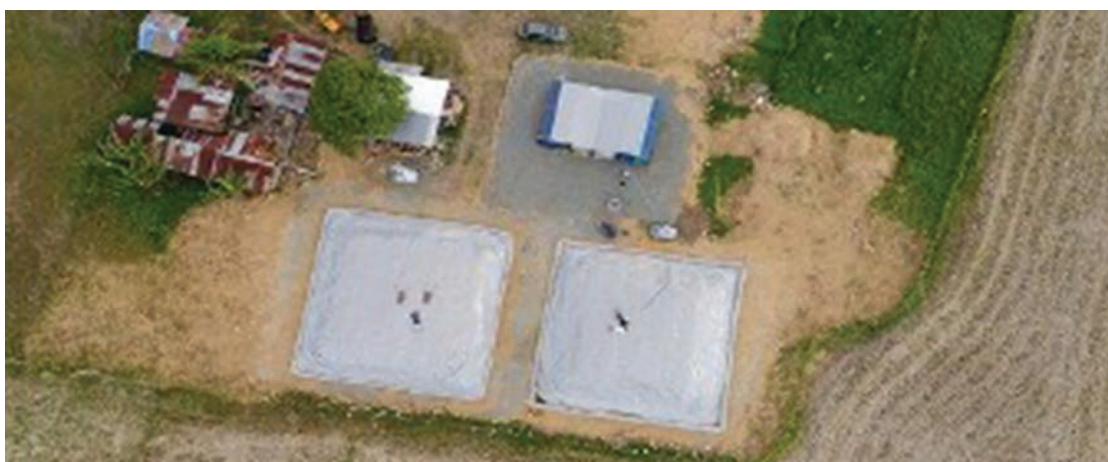
FIGURE 15: Overhead view of a dryQUBE installation in the Philippines
