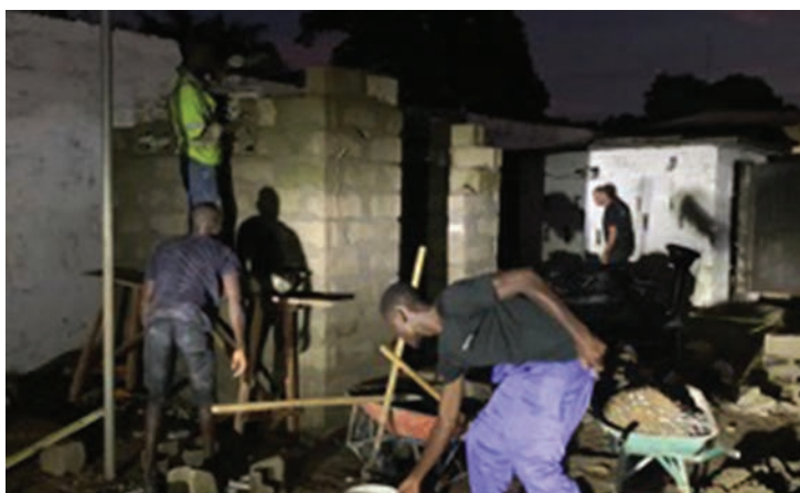
Construction of toilet building at Isaac A Davies School under tight timeframe
