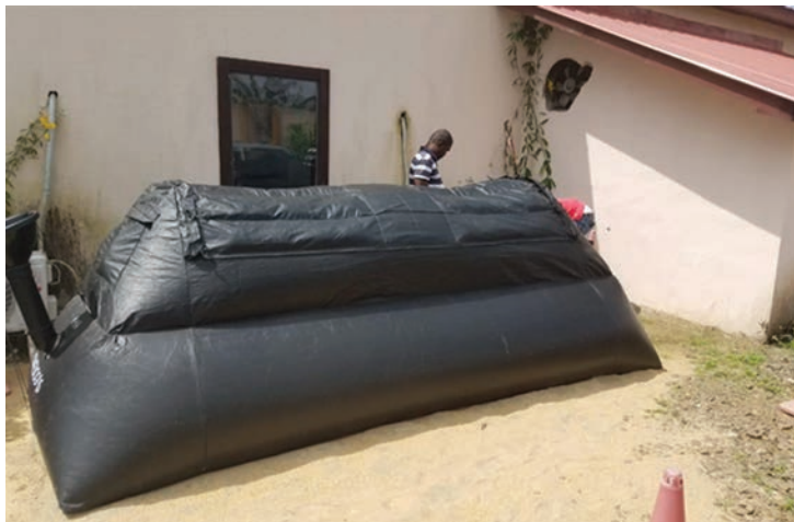
HomeBiogas 7.0 (larger unit) installed at RLJ Kenedja Resort
