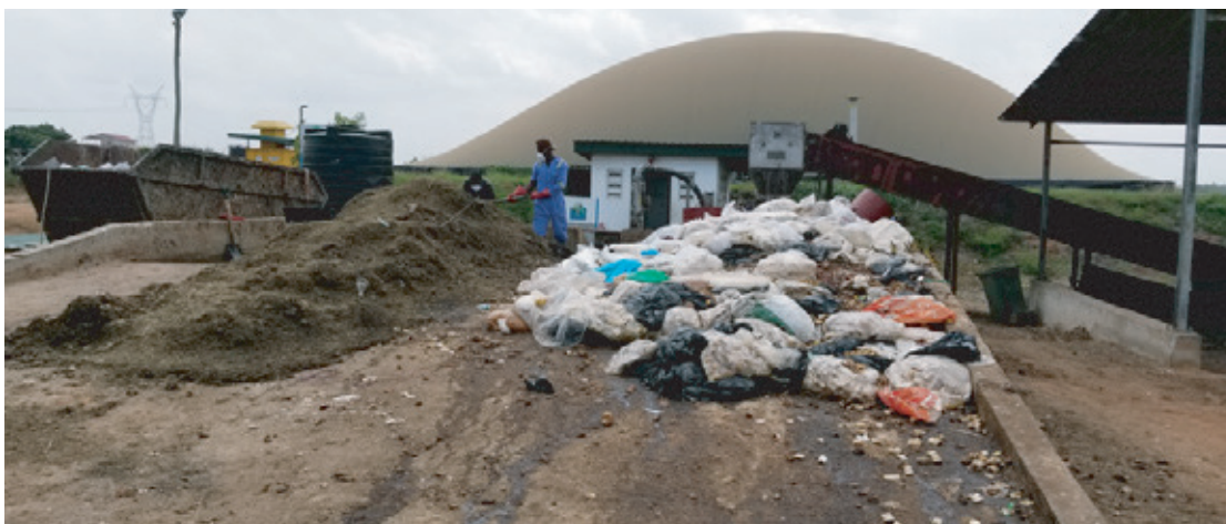
FIGURE 80: Waste-receiving area with digester behind at Safi Sana W2E facility in Ghana
