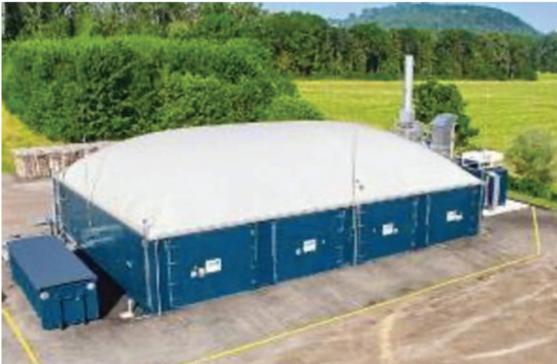
FIGURE 50: BEKON MINI rated at 4,500 tonnes per year of waste organic capacity
