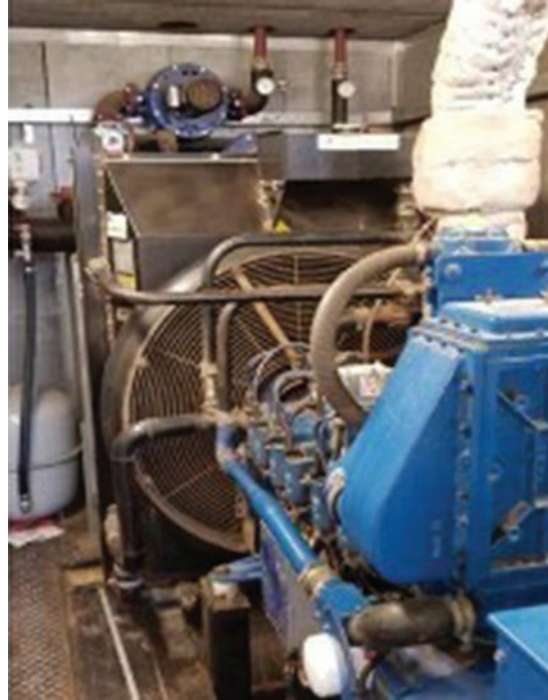
FIGURE 45: Biogas engine generator
