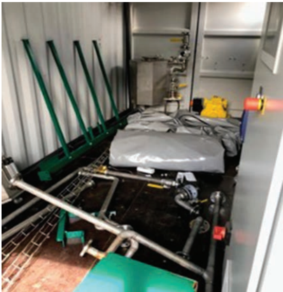
FIGURE 20: bioQUBE biogas storage container contents
