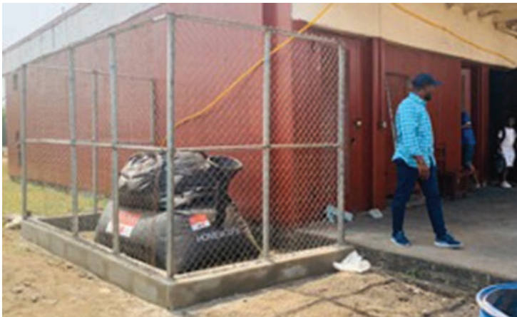
Fence installed at William V. S. Tubman High School
