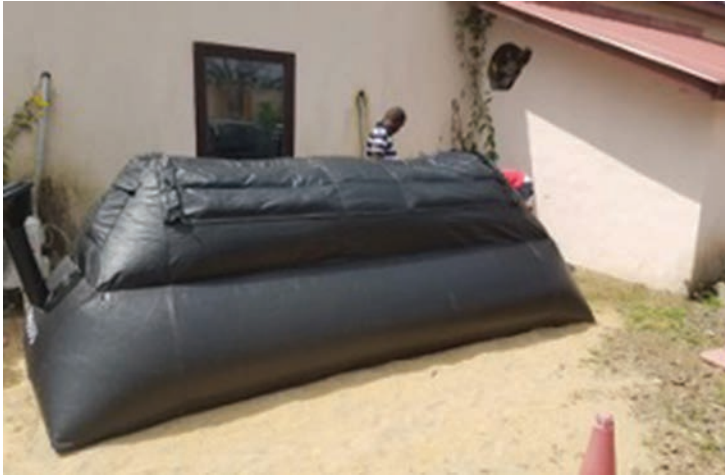
Methane gas production at top of unit being observed
