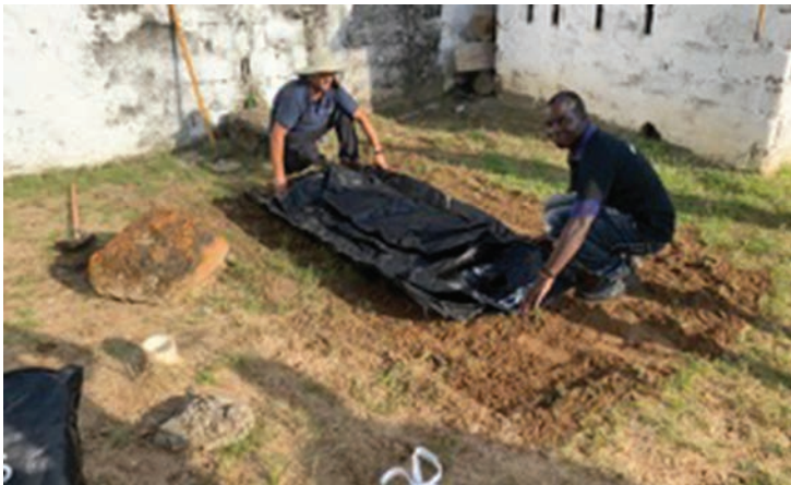
Installing 2.0 unit at Isaac A. Davies School
