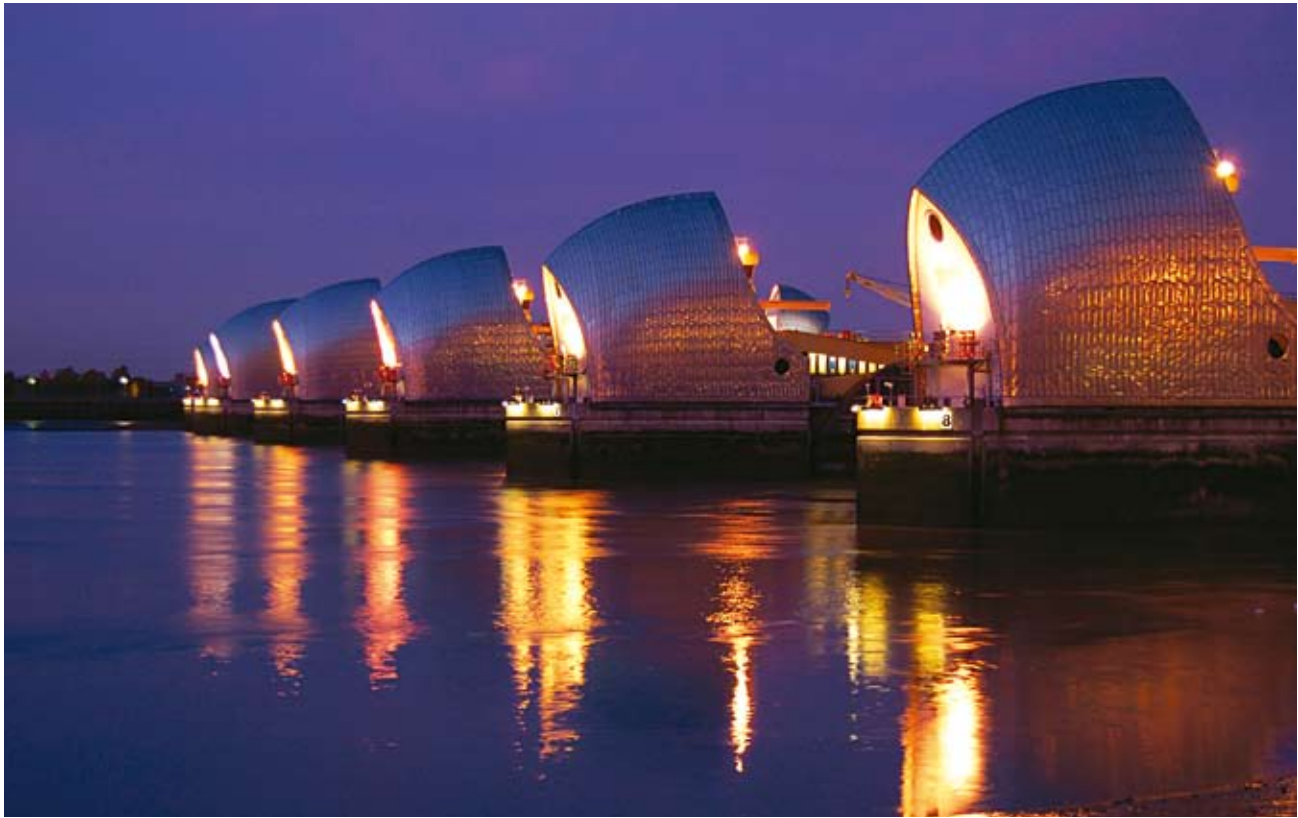
▲ The Thames Flood Barrier, London's first line of defence against floods. ©Adrian Dracup/iStockphoto
