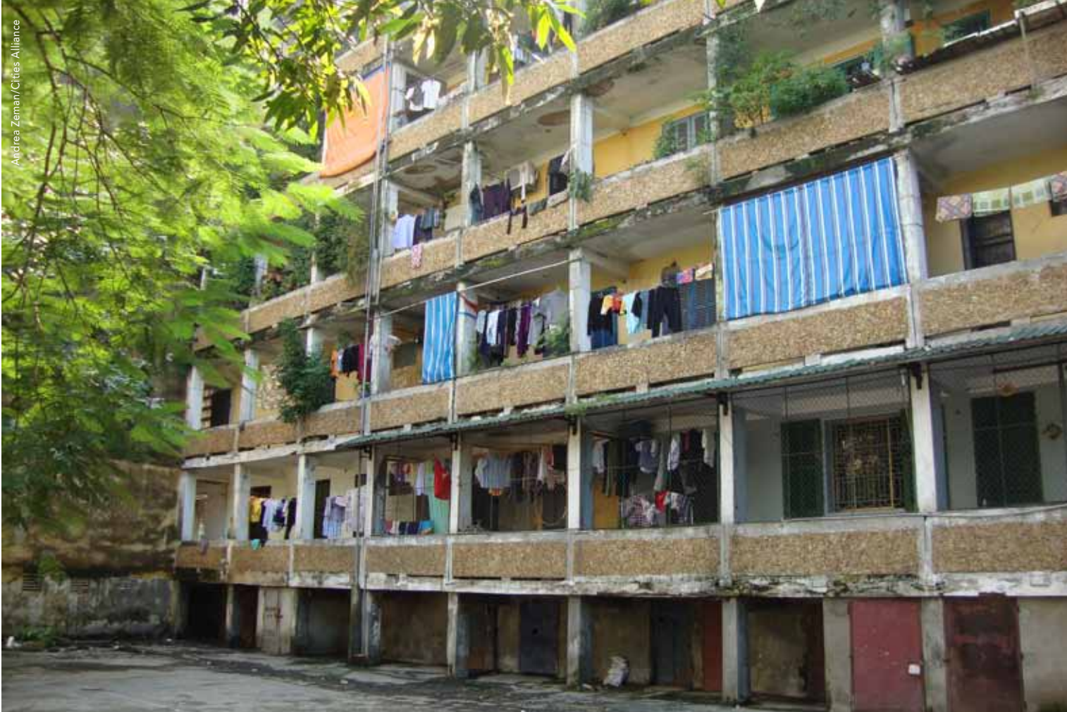
Dilapidated housing in Vinh, Vietnam.
