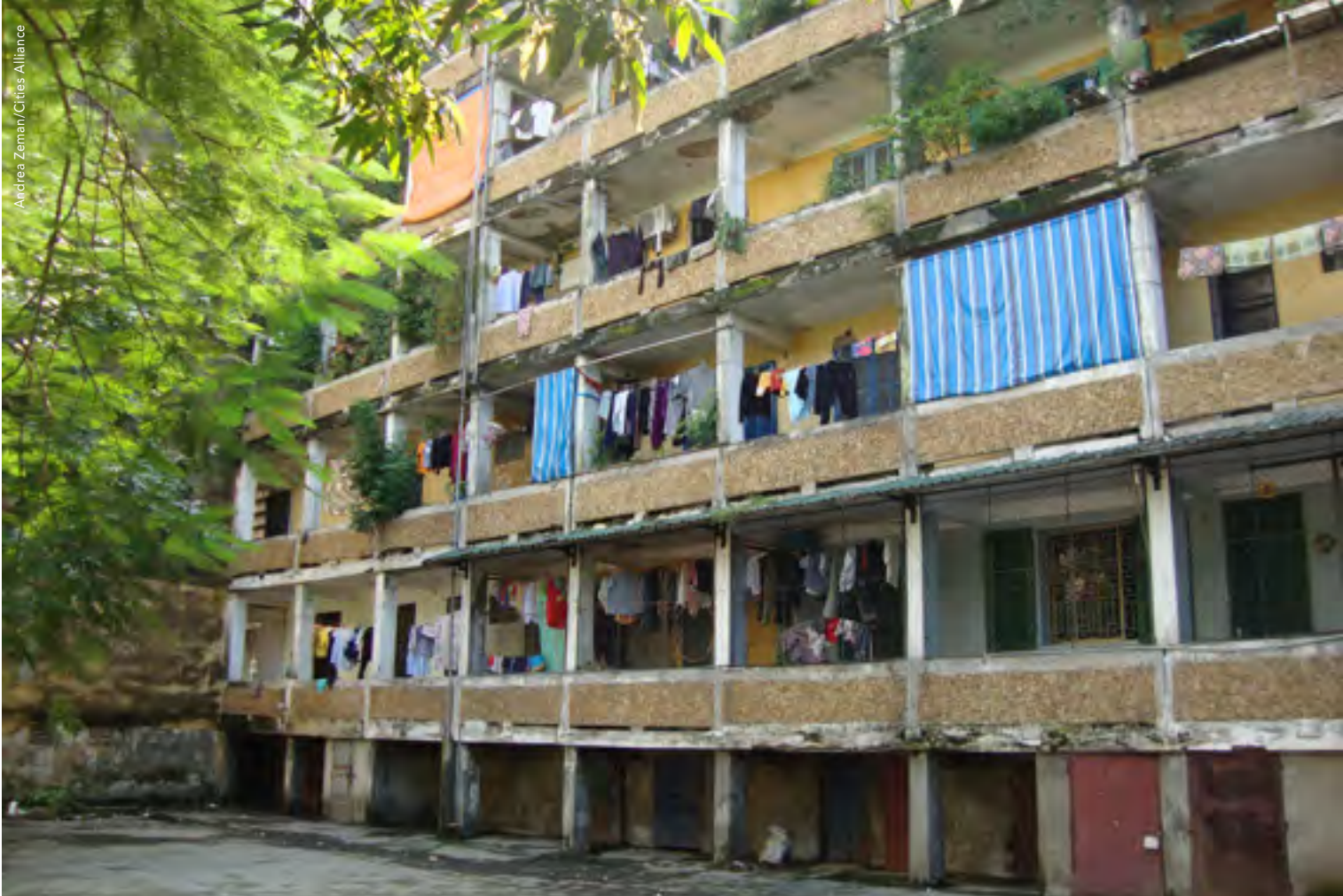
Dilapidated housing in Vinh, Vietnam.
