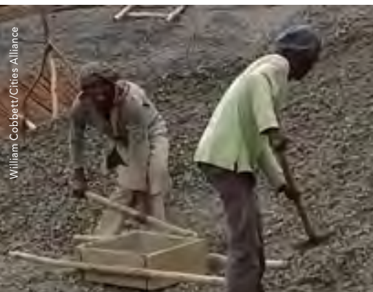
Ethiopia has undertaken a bold housing programme that relies on labour-intensive delivery with limited use of machinery.
