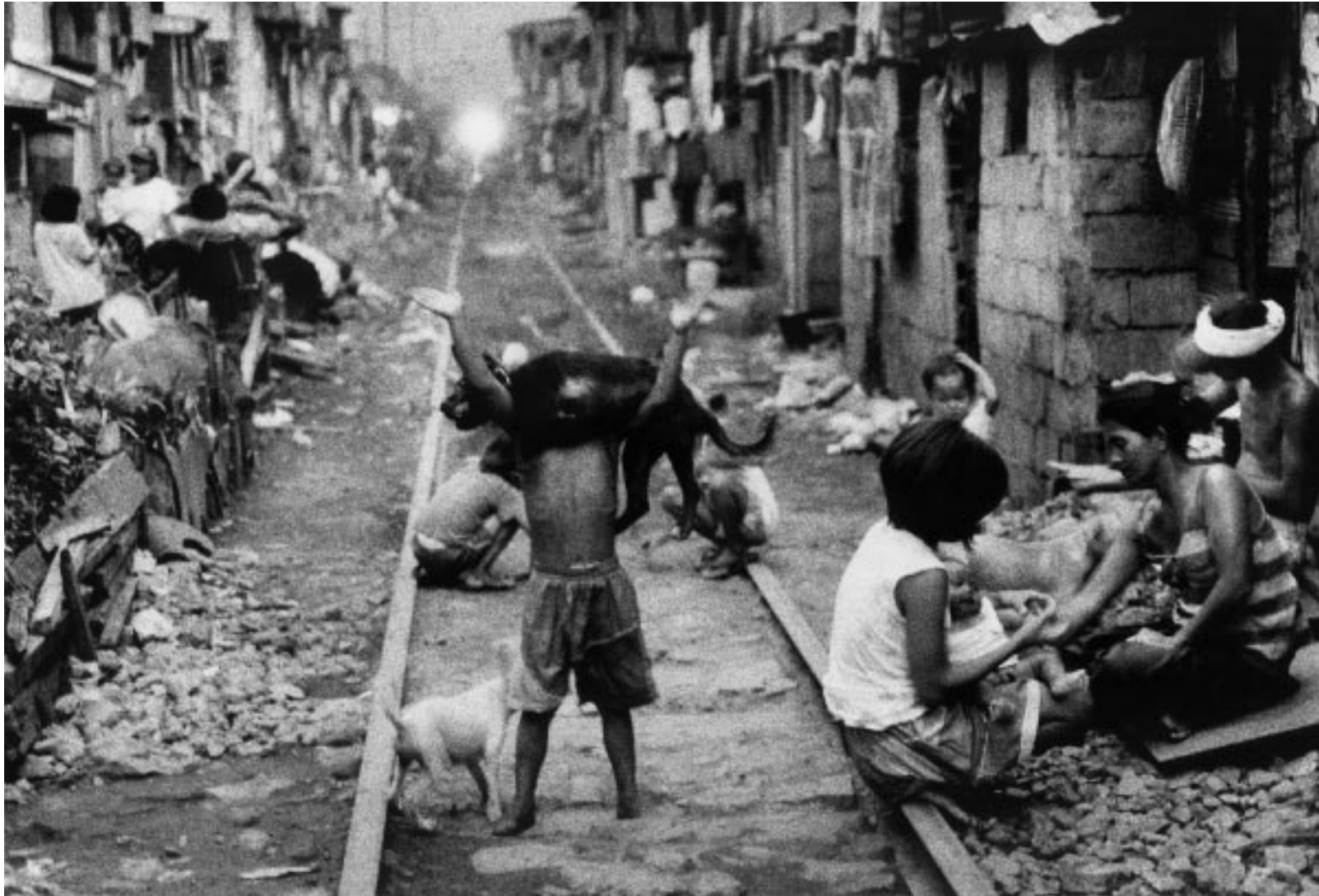
Railroad track through Manila is lined with shacks housing tens of thousands of squatters. Metro Manila, Philippines, 1999.
