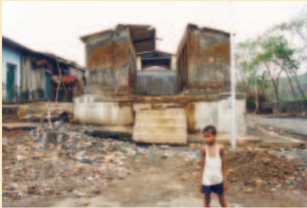
A public toilet, India
