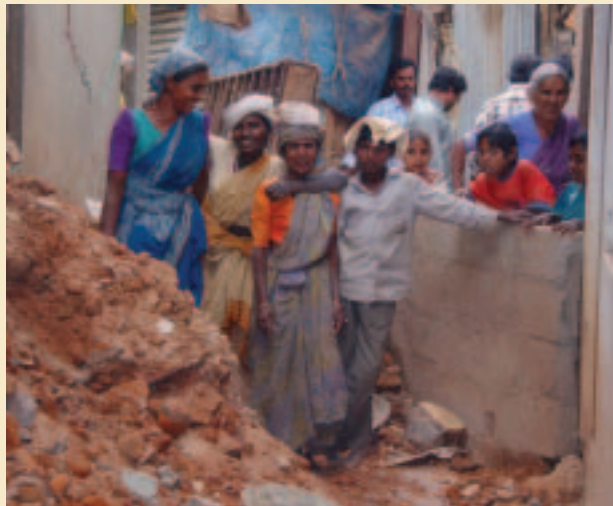
Community members involved in constructing the third housing block at Sunnuduguddu, Bangalore, India. The development at Sunnuduguddu is supported by the CLIFF programme.
