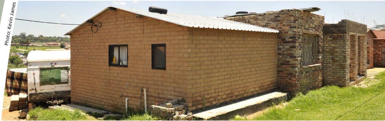
Additions to an RDP house, with caravan accommodation on the left
