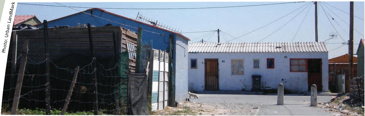
A shack in the yard of an RDP house in Delft
