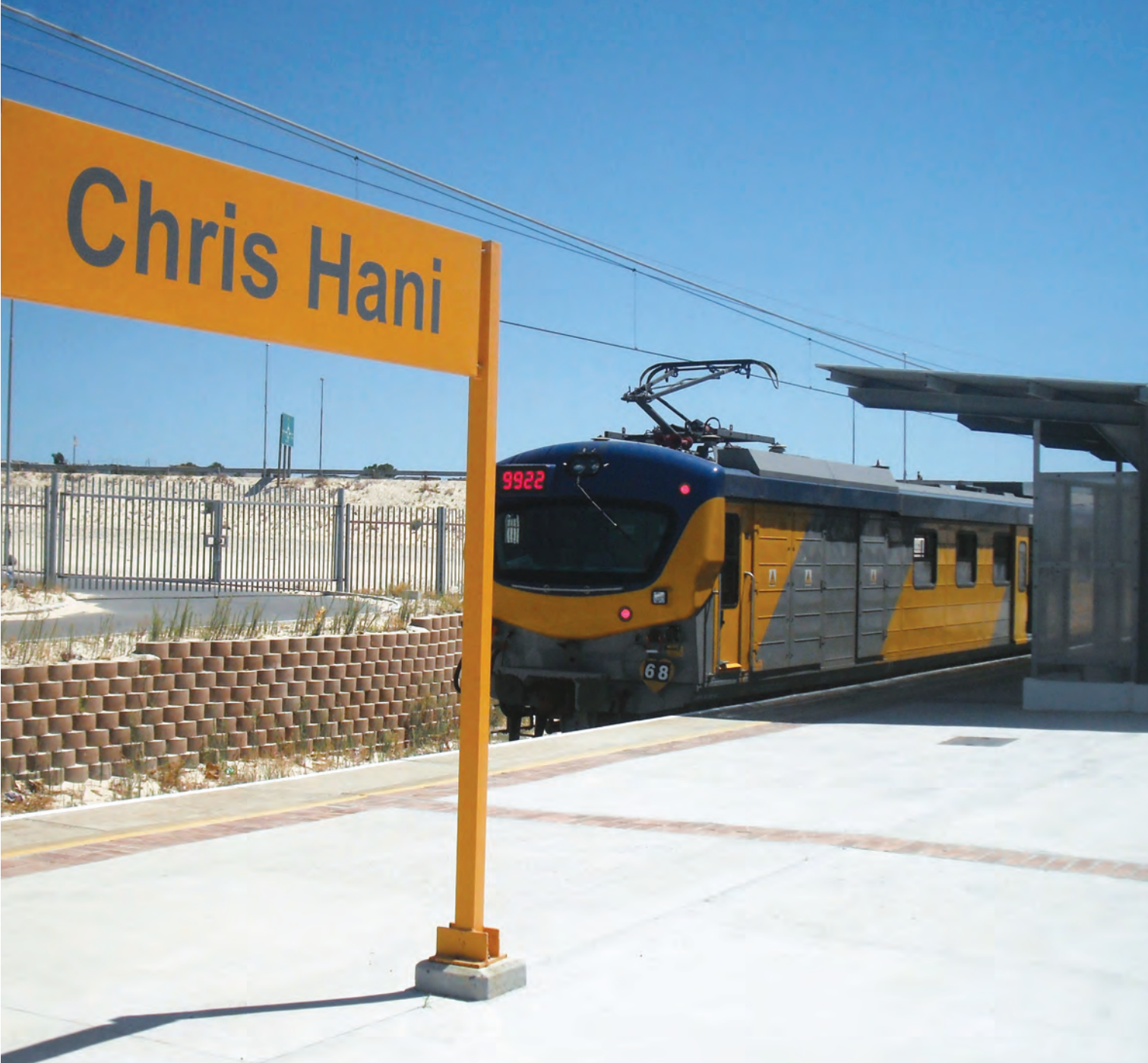
Chris Hani metrorail station in Khayelitsha, Cape Town
