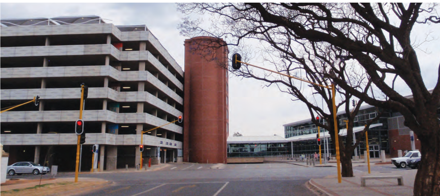
Gautrain station in Hatfield, Tshwane
