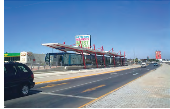
A Bus Rapid Transit station in Soweto, Gauteng
