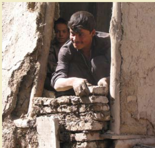
Rebuilding in Afghanistan
